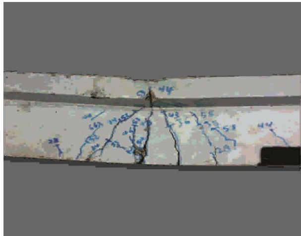
Fig.5 Cracks pattern of beam B4
