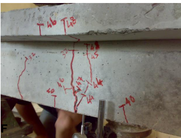
Fig.2 Cracks pattern of beam B1
