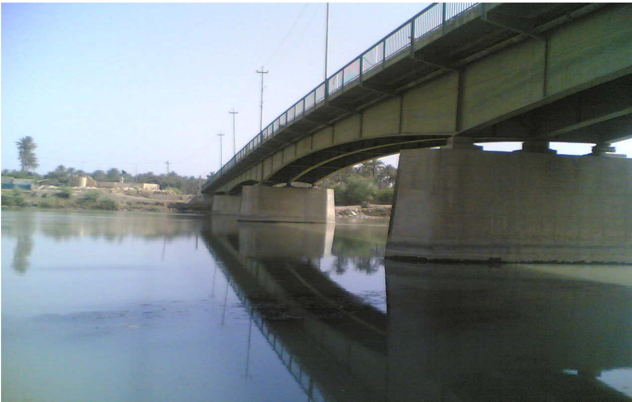
Plate 1. Al – Kufa bridge at Al-Najaf city
