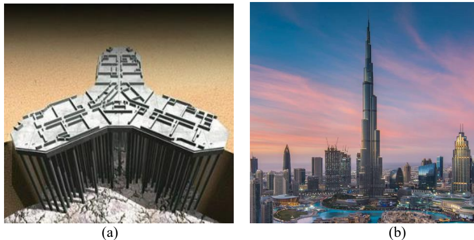
Fig. 1. Burj Khalifa: (a) Foundation system raft shape with supported piles, (b) Burj Khalifa Skyline (El Gendy et al., 2018; Peirce, 2023)
