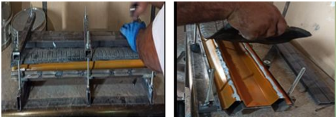
Fig. 2. Steel frame and epoxy for the SUT fixing process.
