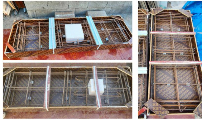
Fig. 6. Molds and Arrangement of steel reinforcement
