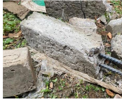
Fig. 2b. Steel reinforcement for ion penetration test
