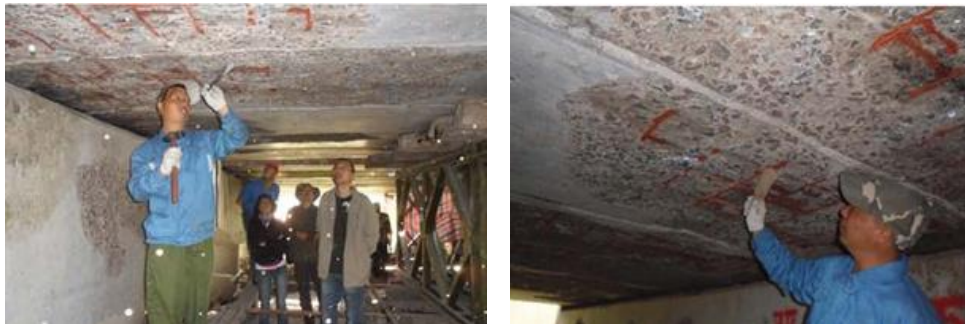
Fig. 4. Cleaning the substrate surface of girder (loose concrete and rusty steel bars).
