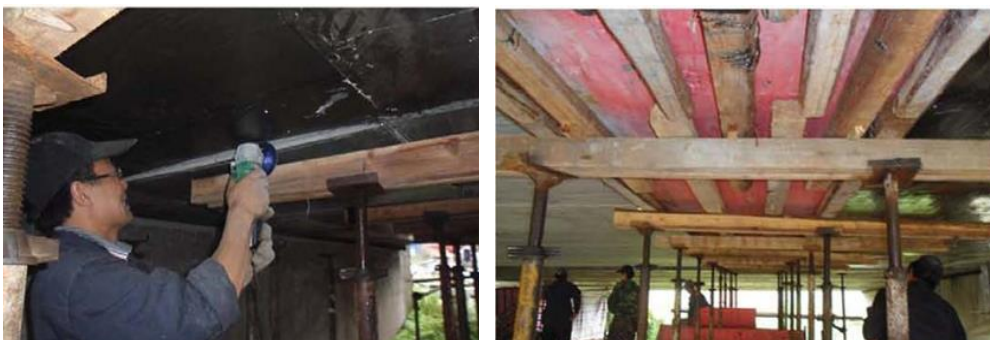
Fig. 5. Fixing Frame and pouring of PUC material.
