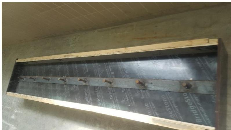
**Fig. 3. Instillation of stud shear connection.**
