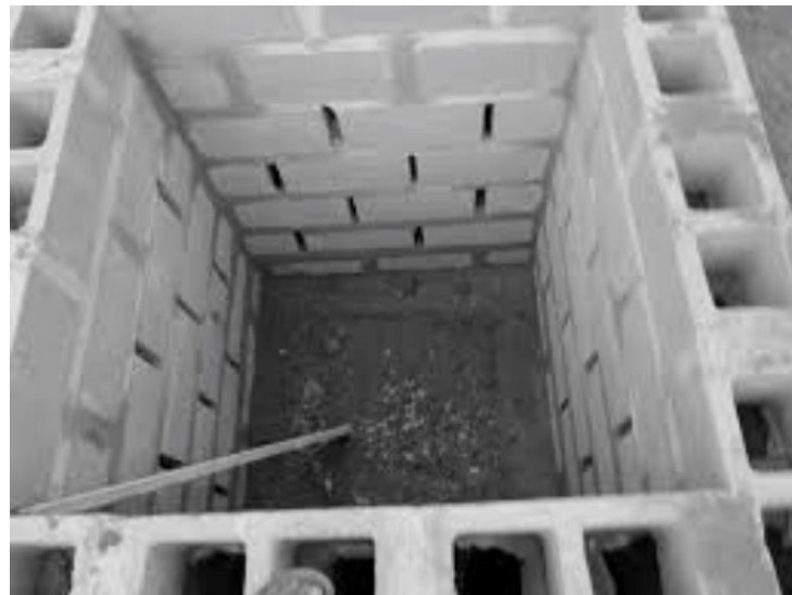
Fig. 1. A typical soakaway construction in Lagos.
