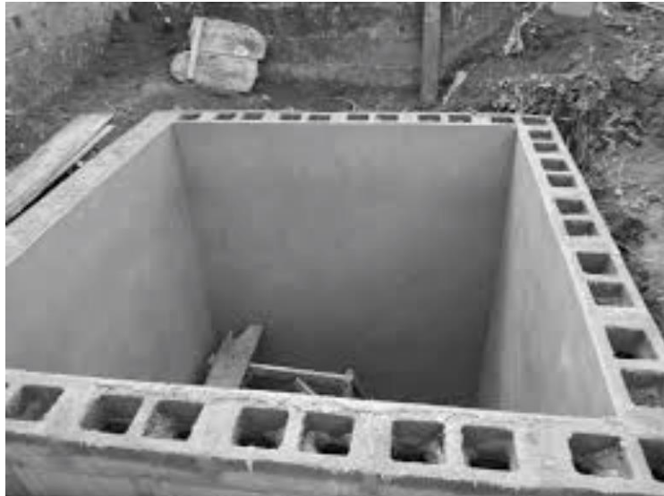
Fig. 2. A typical Septic tank construction in Lagos.
