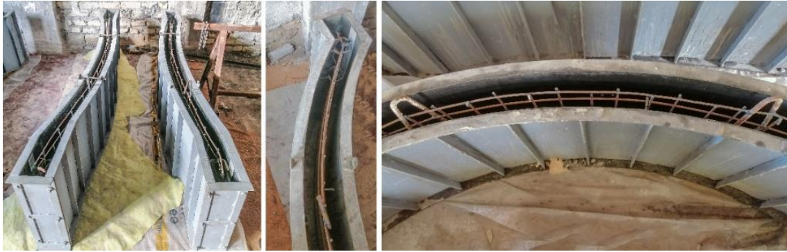
Fig. 3. Reinforcement of the Samples.
